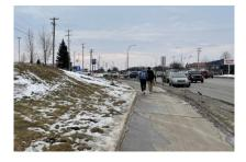
Sidewalks: A concrete path (minimum 4' width, 5' preferred, 6' ADA compliant)
