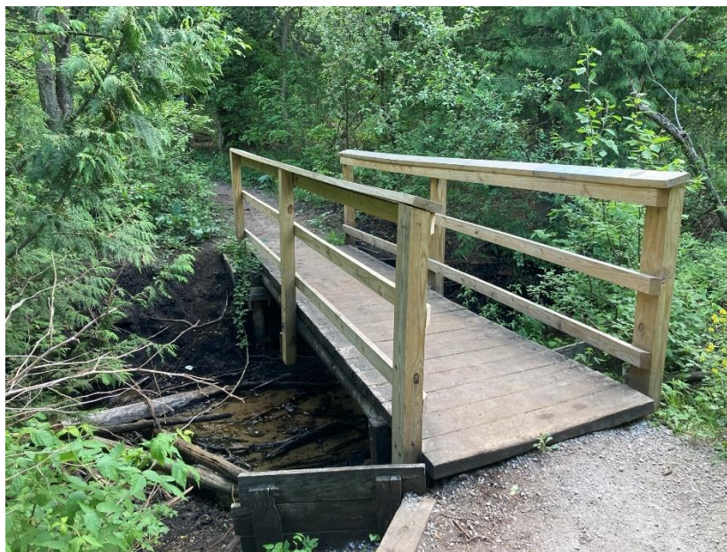
Footbridge in the Commons Natural Area (Photo: May 2021)
