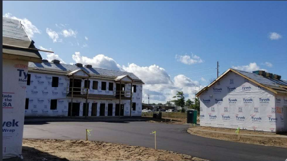
New housing construction - Aspen Pines on Floresta
