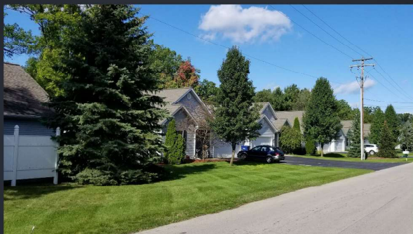
Recent housing construction - Duplexes on Woodward
