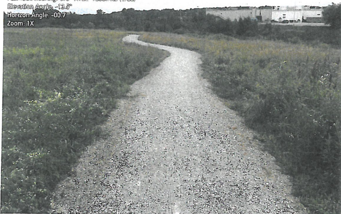
Facing NE along the new trail from its south end near the south boundary of the property and its intersection with the paved trail from the YMCA.
