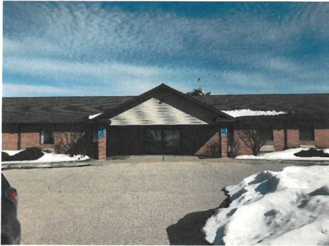
West side of building.
