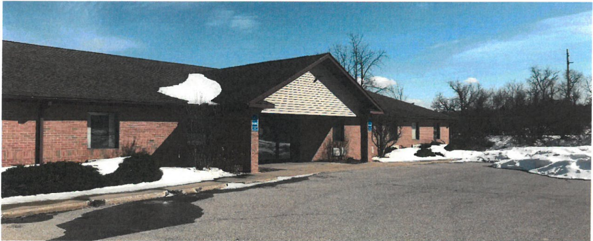
Front entrance. West side of building.
