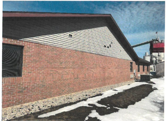
South side of building.
