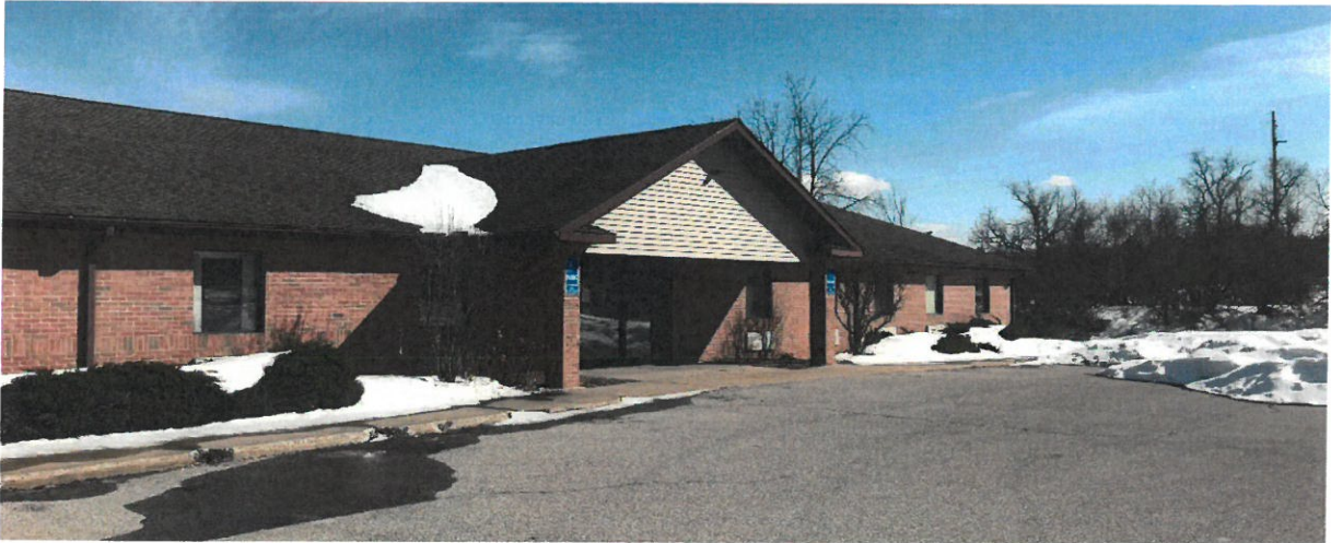
Front entrance. West side of building.
