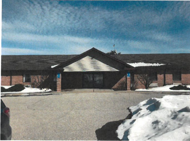
West side of building.
