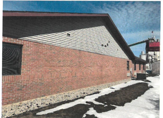
South side of building.
