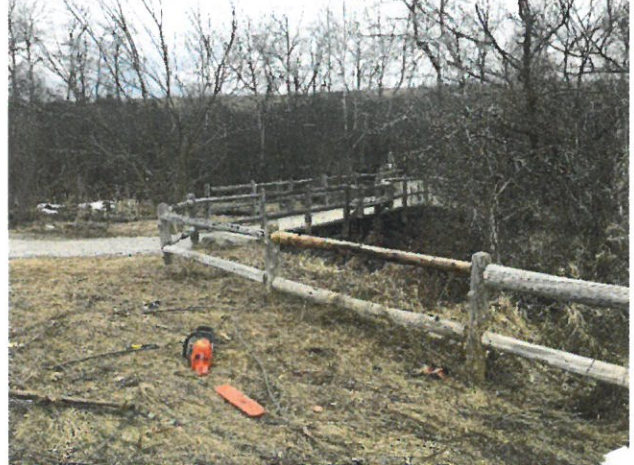
Fencing Rail Replacement along Kids Creek
