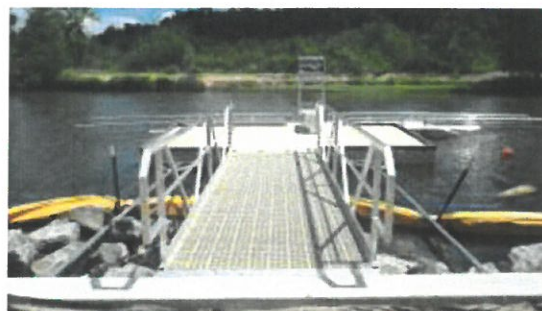
Universally accessible boat launch installed
