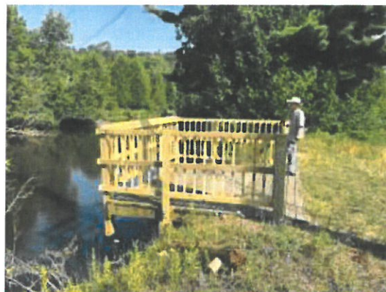
Railing replaced on viewing/fishing platform
