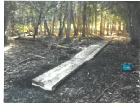
Cedar Cathedral Boardwalk Extension
