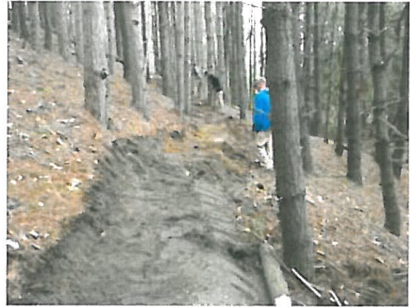
Bench trail construction at Miller Creek NR
