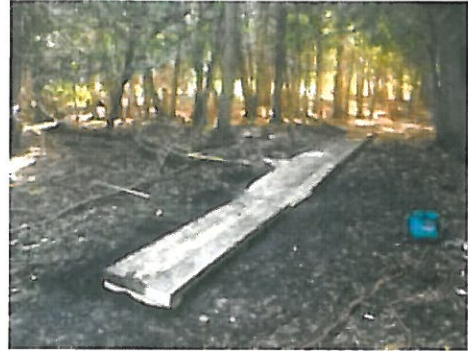
Cedar Cathedral Boardwalk Extension
