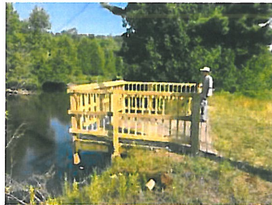
Railing replaced on viewing/fishing platform
