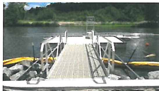
Universally accessible boat launch installed
