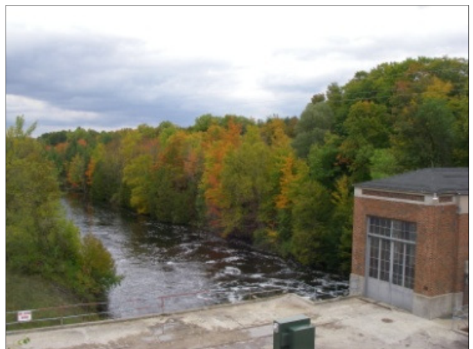
The removal of three dams on the Boardman River, two in Garfield Township, will allow the river to return to a more natural state as a free-flowing, cold-water river. This project is the largest dam removal project in Michigan's history and the largest wetlands restoration in the Great Lakes Basin.
